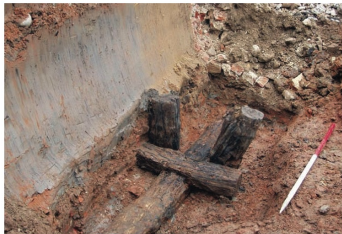
Below These timbers supported the wall of the dock during construction.
